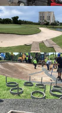
A minimum of eight pieces of 4" (100 mm) to 6" (150 mm) diameter irrigation or drainage pipe cut into 2 inch (50 mm) lengths. Use these rings to maintain the 2 inch (50 mm) required minimum depth of the Capillary Concrete during placement. Remove the rings from the wet mix as you work out of the bunker. Attach a handle or make a wire loop on each piece of pipe to avoid losing them in the mix. A metal probe set at 2 inches (50 mm) is also acceptable.
