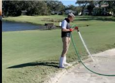
It is recommended that a tracer wire be installed in all drainage trenches. The drainage pipe must be flushed with plenty of water to ensure proper function prior to installation of Capillary Concrete in the bunker.
