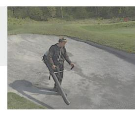
Now perform the water drainage test to confirm that water rapidly drains through the product. This must be done to activate the Performance Guarantee. Do not "blast" high pressure water on the freshly installed Capillary Concrete - a shower spray is preferred over a steady stream. **See the film: The Test of Drainage.**
